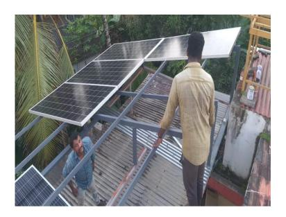
Fig: 62. Solar panel installation
